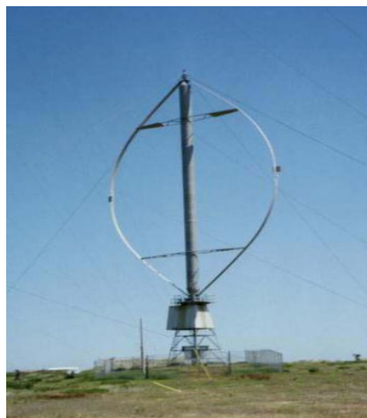
Figure 12: VAWT (Darrieus type) for electricity generation
